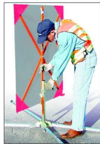
Rectangular signs need third vertical rib to secure to stand, and flex during wind gusts
